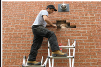
All Brick Work & Repairs
