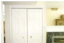
Doors, Flooring, Trim
