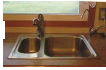
All Plumbing & Fixtures
